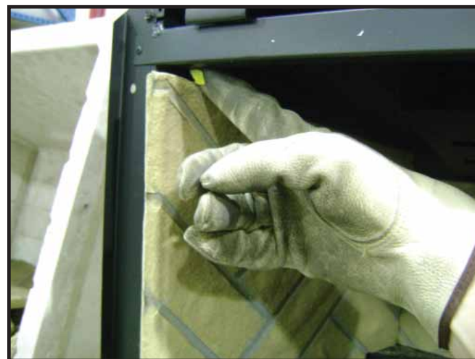
Figure 5. Bend Refractory Tab
