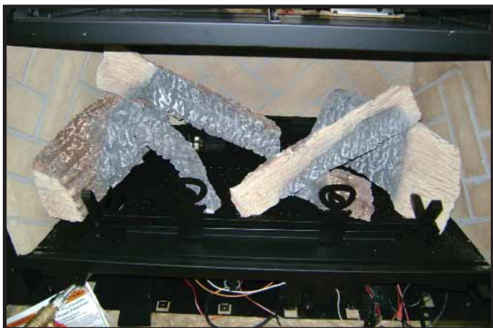
Figure 2. Refractory and Logs Installed
