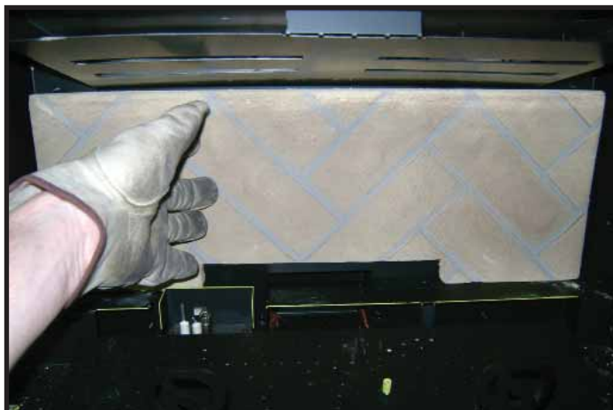
Figure 3. Install Back Refractory
