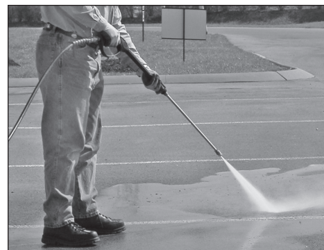
Figure 14 - Optimum angle to cleaning surface
