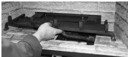
Diagram 1: Remove the left and right screws and then slide the burner/grate assembly to the left and lift out.
