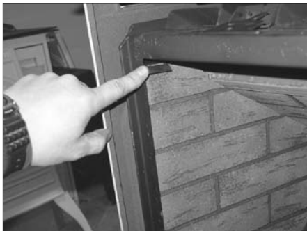
Figure 8.17 Bend over tabs to hold panel in place.
