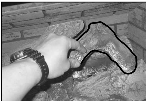
Figure 8.23 Place right twig over the locator pins on the rear log and the right front log.
