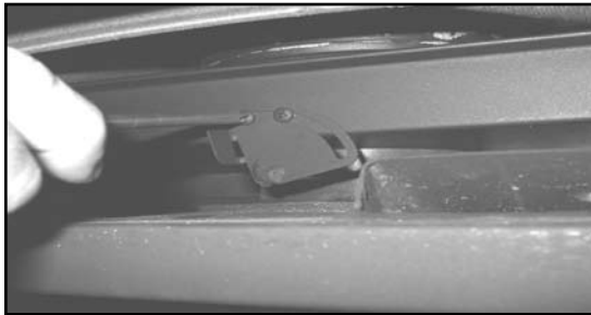
Figure 8.32 TOP VENT INSTALLATIONS: Locate the damper adjustment on the intake plenum. Access through the appliance front. Adjustor is centered at the top of the appliance.
