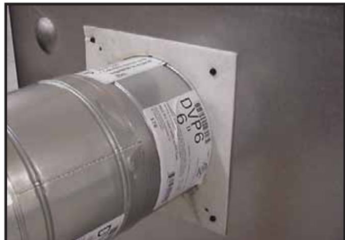
Figure 9.12 Attach the first vent section (it will snap into place). Slide the insulation gasket onto the vent section, up against the appliance and over the tabs. Use two self-tapping screws to secure gasket to outer wrap.
