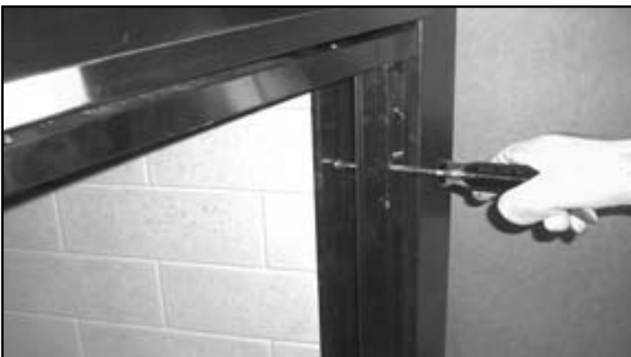
Figure 11.3 Loosen Refractory Retaining Strip
