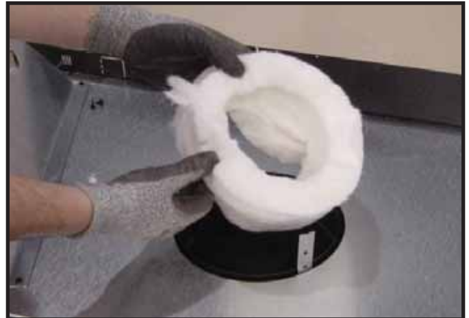
Figure 9.5 Remove the insulation from the outer vent pipe. For rear venting there is no insulation in the outer vent pipe.
