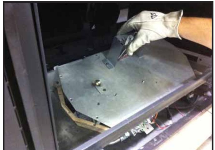
Figure 11.3. Remove Valve Plate
