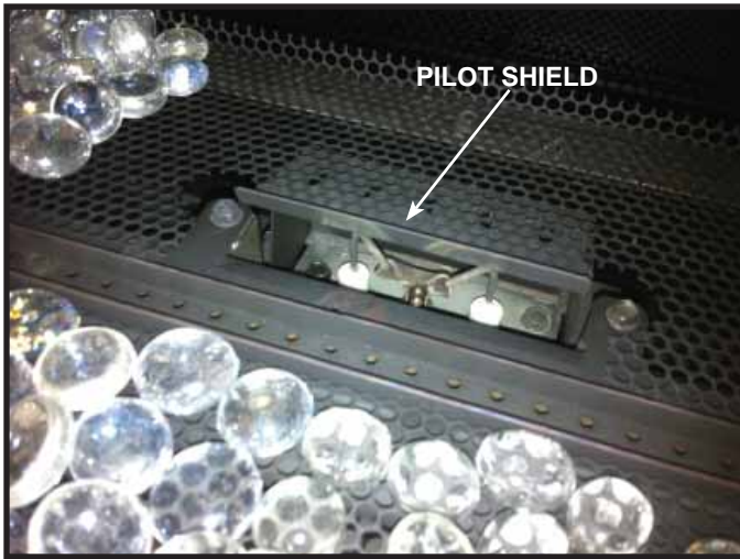
Figure 14.3. Placing Glass Rock Media on Pilot Shield
