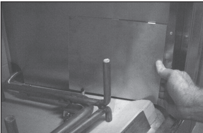
Figure 6.3 Remove Valve Access Panel
